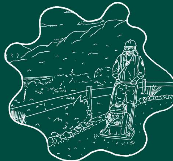
Park ranger compacting a bushwalking track
